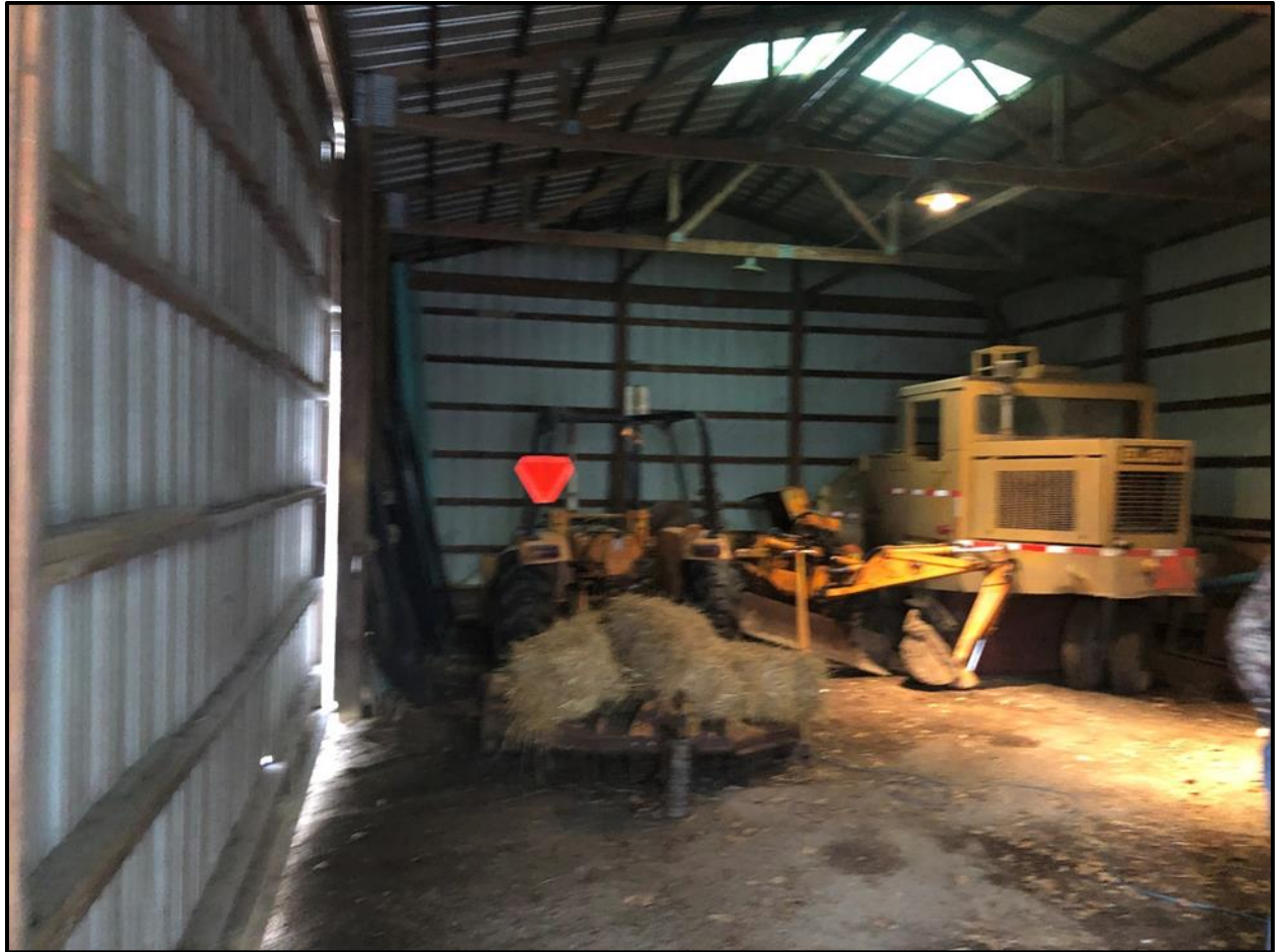
Figure 4 – East vehicle bay (standing west looking east).
