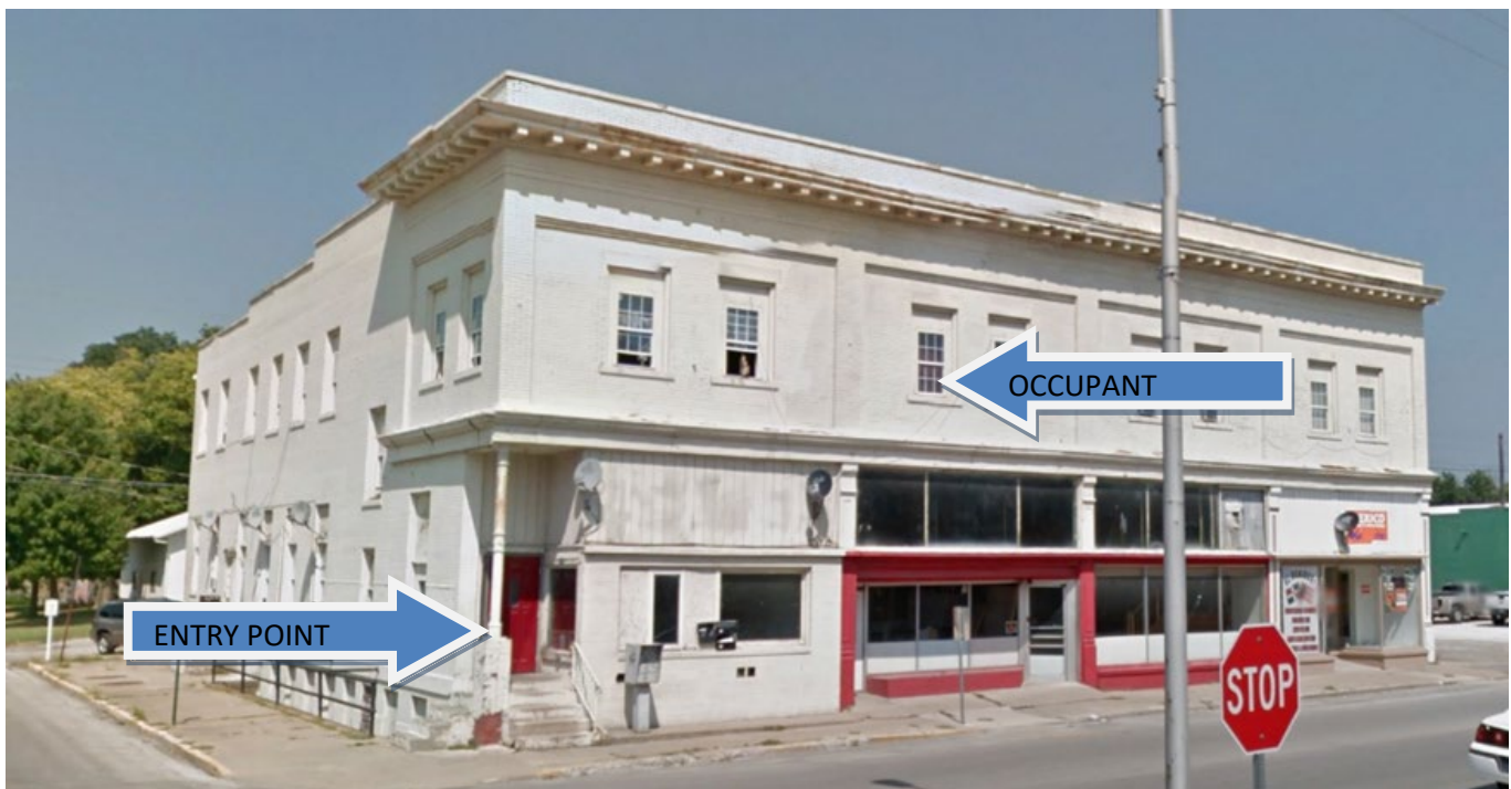
Figure 4 – Alpha/Bravo side of building (photo credit: Google).
