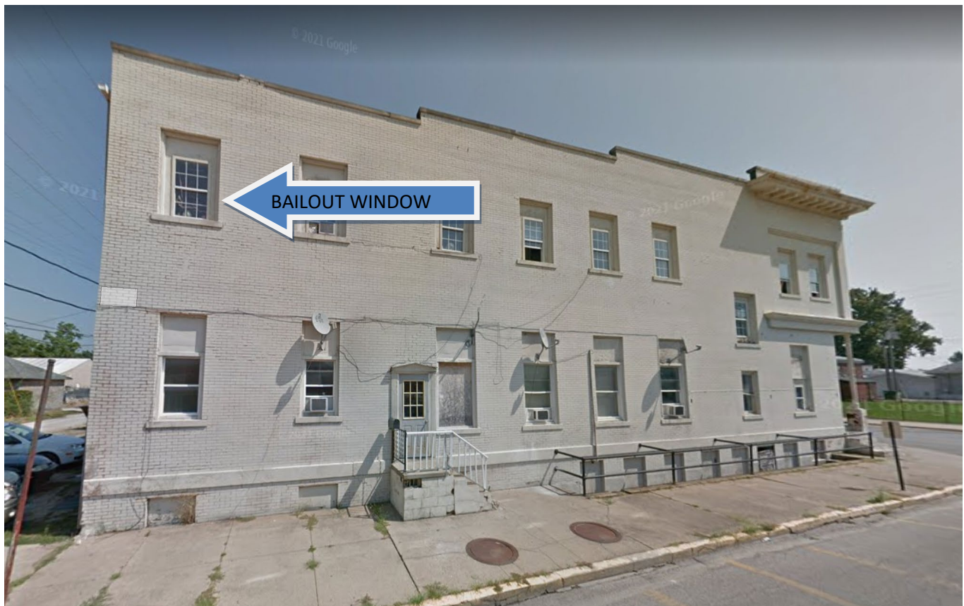
Figure 5 – Bravo side of building (Photo credit: Google).
