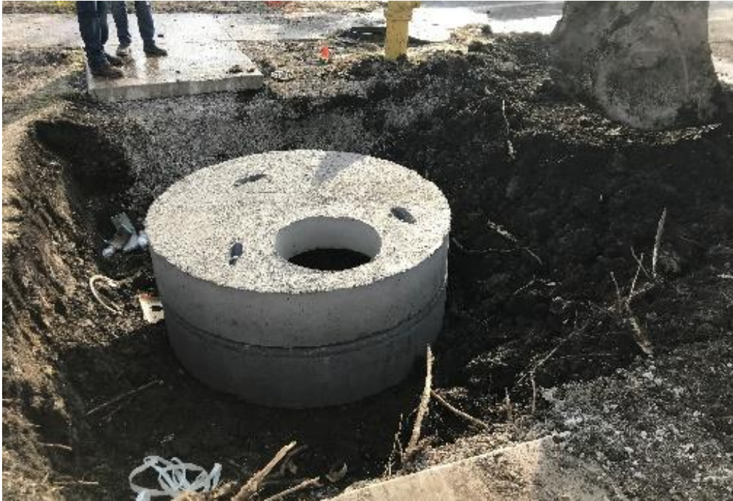
Figure 10 – Valve vault after excavation, post-incident.
