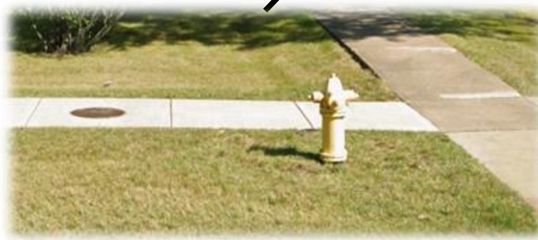
Figure 1 – Street map of area with photo of worksite. Manhole cover (above left) provides access to valve vault. (Photo credit: google earth)
