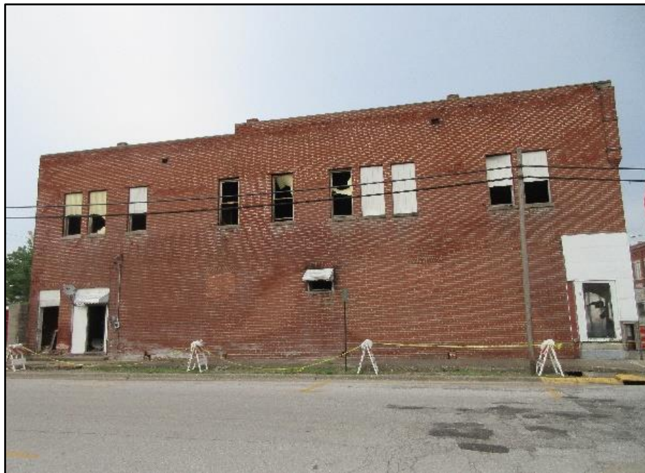
Side Bravo of the fire building. (NIOSH photo)
